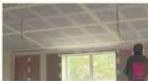
PLASTERBOARD STOPPING
