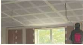
PLASTERBOARD STOPPING
