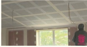
PLASTERBOARD STOPPING
